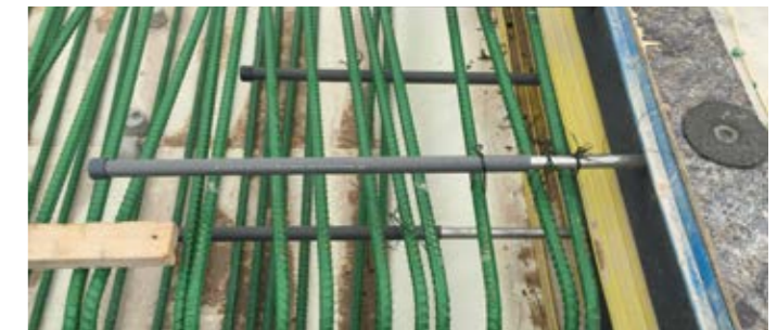
Mega Reservoir project, Qatar
