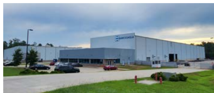
Richburg bar finishing mill
