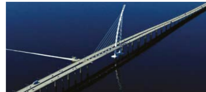
Sheikh Jaber al-Ahmad Al-Sabah Bridge, Kuwait
