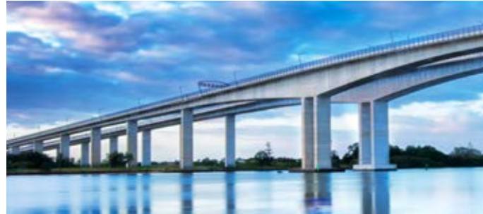
Gateway Bridge, Brisbane, Australia
