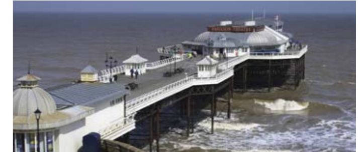
Coast protection scheme, Cromer, UK
