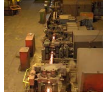
Rolling A highly responsive digital control system tracks the rod through the mill to ensure quality.
