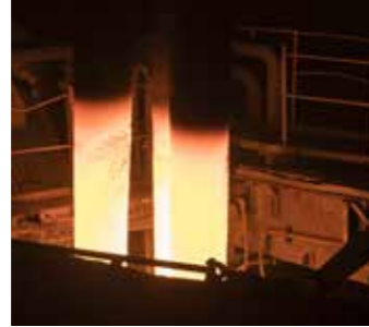
Electric arc furnace The 130 tonne, 90 MVA furnace melts the stainless scrap into a liquid feedstock.
