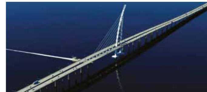
Sheikh Jaber al-Ahmad Al-Sabah Bridge, Kuwait
