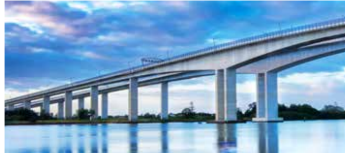
Gateway Bridge, Brisbane, Australia
