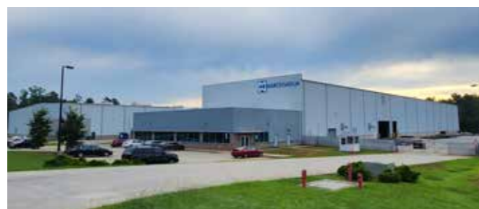
Richburg bar finishing mill
