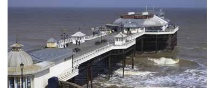
Coast protection scheme, Cromer, UK
