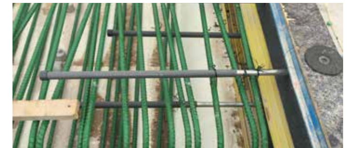
Mega Reservoir project, Qatar
