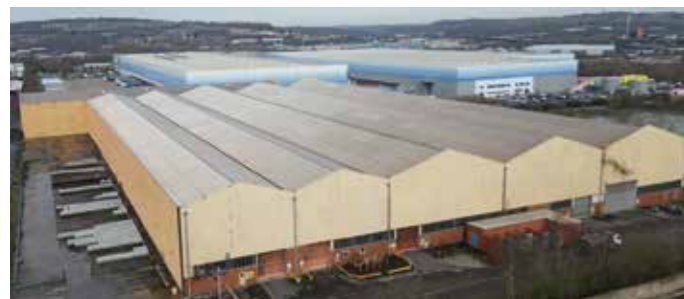
SSB bar finishing mill
